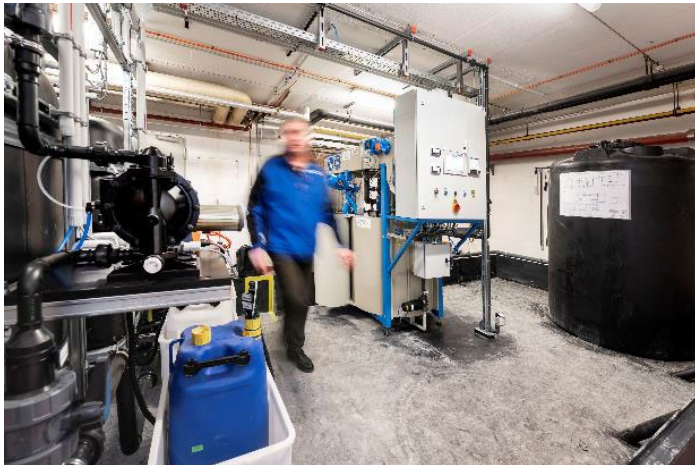
Image: The compact Split-O-Mat SOM 500 unit for treating wastewater generated during production of optical glass
