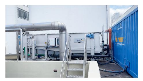
EnviRent rental plant in operation at a dairy, comprising a flotation unit and, on the right, the technical module containing all further wastewater treatment components.
