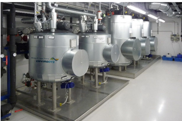
Image: EnviroDTS thermal wastewater disinfection for BSL4 wastewater from the Robert Koch Institute in Berlin
