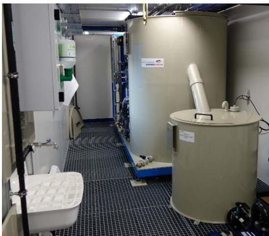
Image: View of the EnviModul plant room with Lugan® 10.000 flotation system for wastewater treatment.
