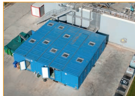
EnviModul plant for decentralised wastewater treatment for cosmetics production in Eastern Europe.
