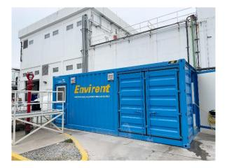
Envirent rental system with an Envochem Ion ion exchange system recycles up to 80% of the water from condensate
