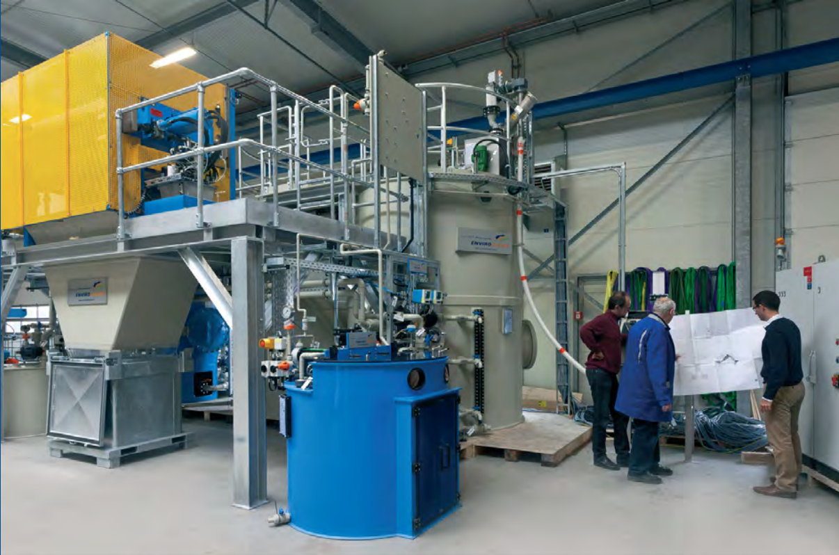
Enviochem® chemical physical wastewater treatment plant ready for FAT
