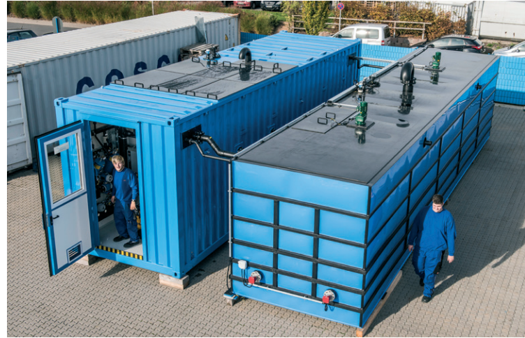
Pre-assembling of an EnviModul modular plant system with Biomar® OMB membrane biology
